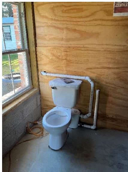
New up flush toilet, installed by Mike Kamansky
