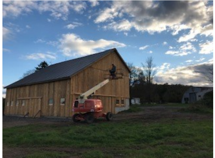
Placing the first of three glass lightening rod balls
