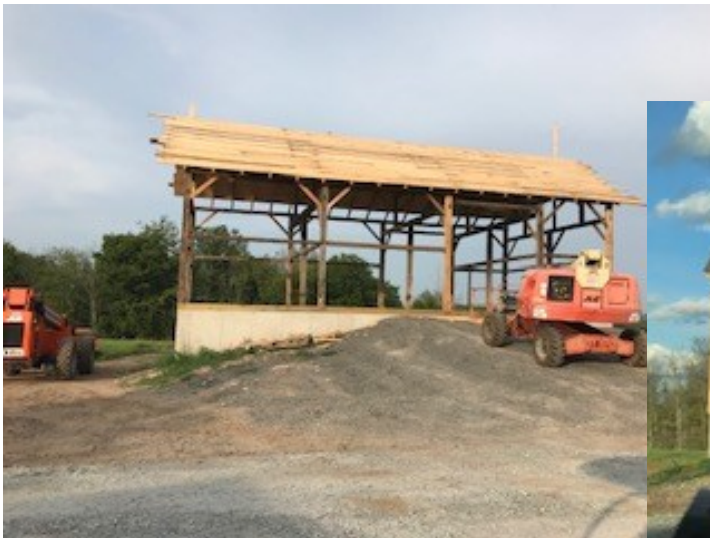
Getting a new roof and life
