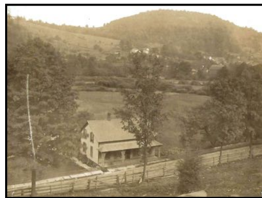
Former Robinson Farm on Brooklyn Road.
