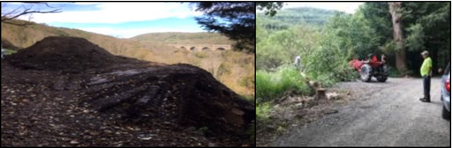
Martins Creek Viaduct scenic overlook site under development
